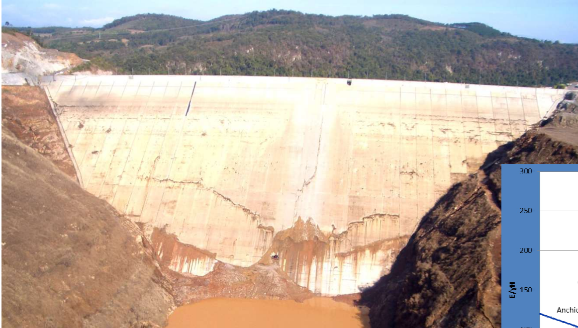
Campos Novos Dam
