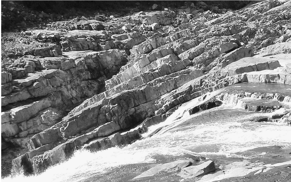
Fig. 10. Erosion at Mokolo Dam spillway, Waterberg Mountains, South Africa.
